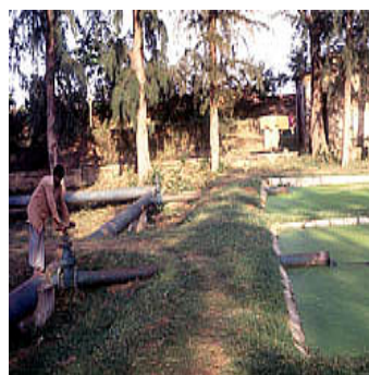
A river of raw sewage (left) runs out of the city of Cuttack. One million litres a day are pumped into an experimental Aquaculture Sewage Treatment Plant (right), where it is treated with aquatic weeds and fish.
