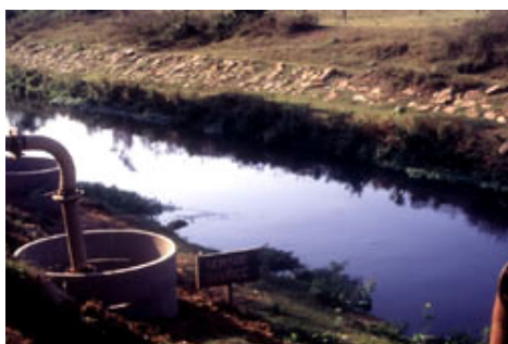
A river of raw sewage (left) runs out of the city of Cuttack. One million litres a day are pumped into an experimental Aquaculture Sewage Treatment Plant (right), where it is treated with aquatic weeds and fish.
